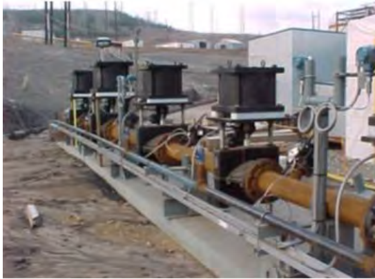
Dropping 250 psi of pressure on a tar sand slurry in Alberta Canada
